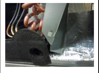
Fig. 9d: Bottom Rail to Outside Support (11U73 shown)
