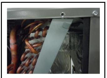
Fig. 9c: Top Rail to Outside Support (11U73 shown)
