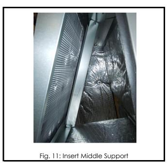
**Step 3** - Insert the second filter, and slide along the track until contract is made with the angled section of the Middle Support.
